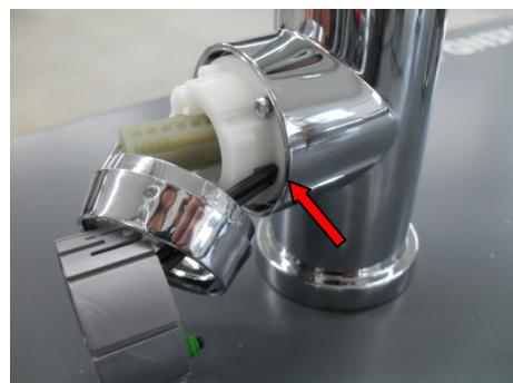
Pull both cables through the hole from the bottom until the shrinking hose sits on the white plastic ring
